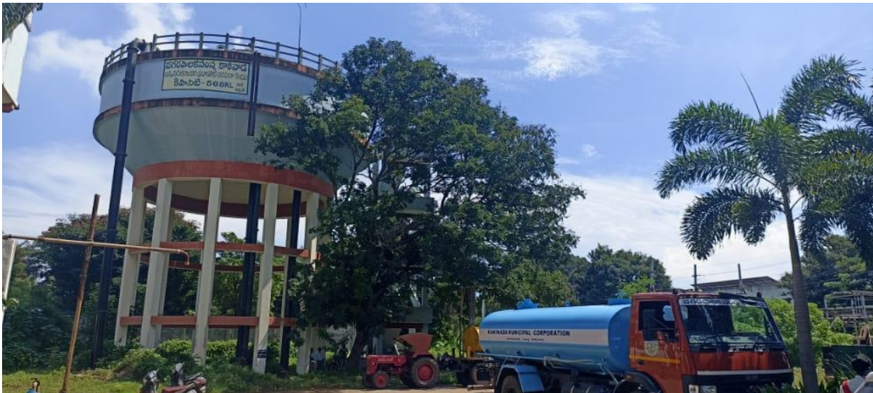
Fig: 9 Filtered water ready for distribution in the city
