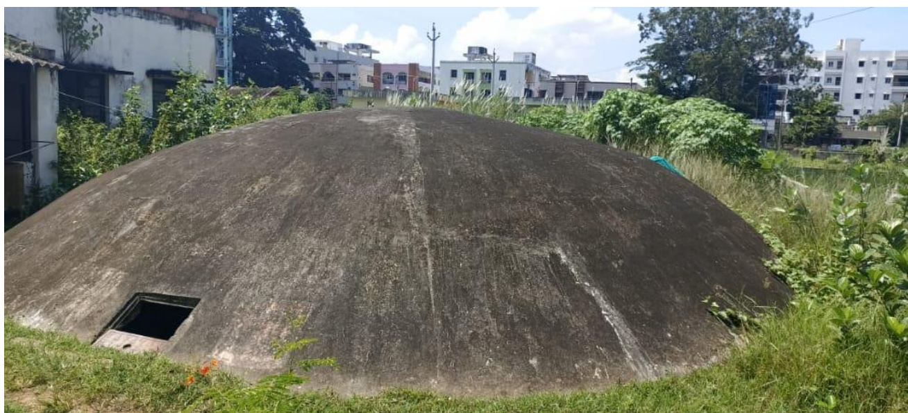
Fig: 8 Chlorinated water stored in the tanks for checking the ppm of Chlorine before supply
